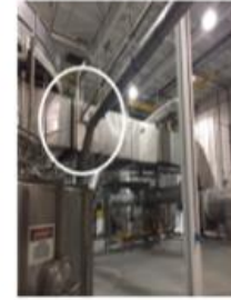
Fig. 17. Example of an interior expansion joint that needs regular inspections
