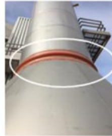
Fig. 16. Example of an exterior expansion joint that needs regular inspections
